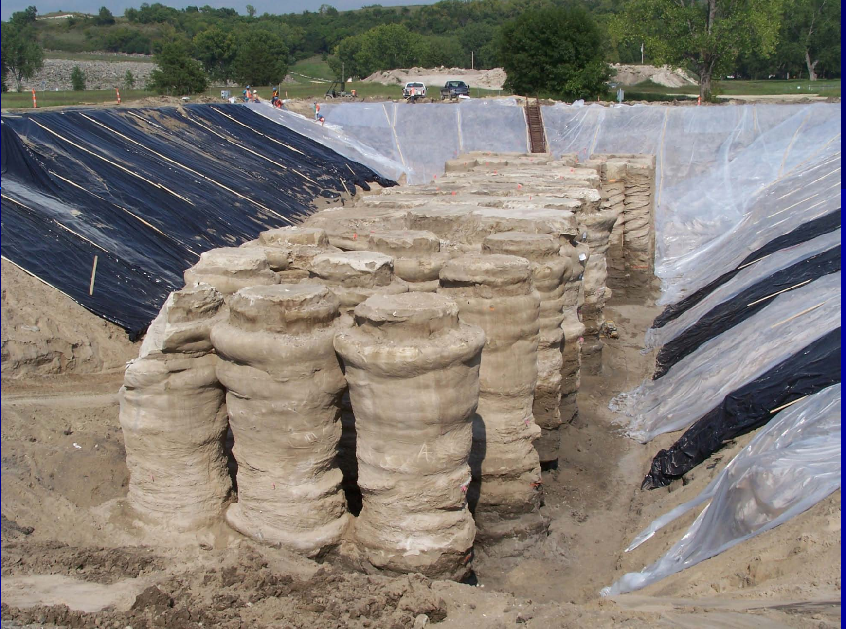
Jet Grout and CDSM Columns at a Recent (2006) Dam Test Section
