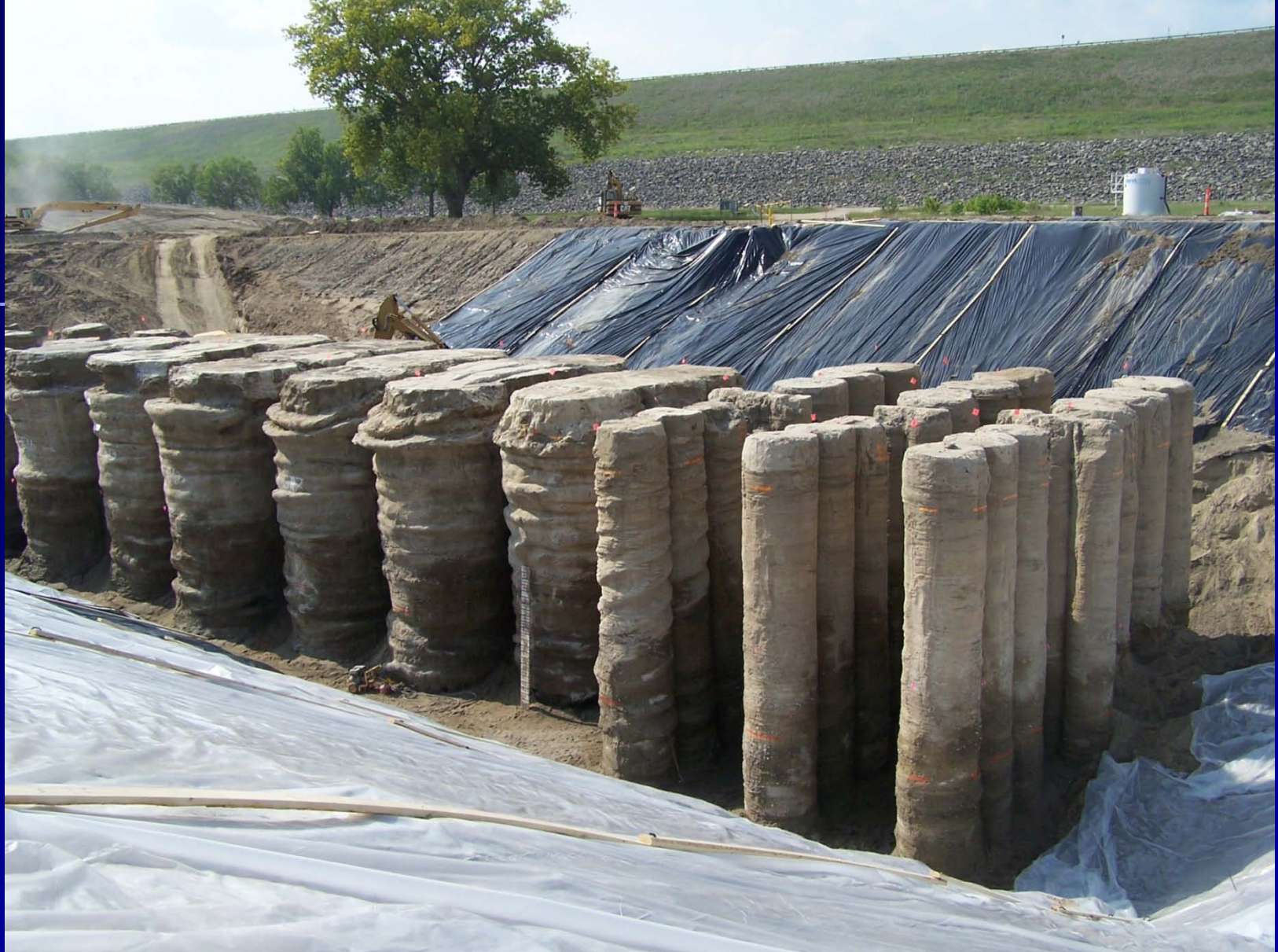
Cement Deep Soil Mix and Jet Grout Columns at a Recent (2006) Dam Downstream Test Section
