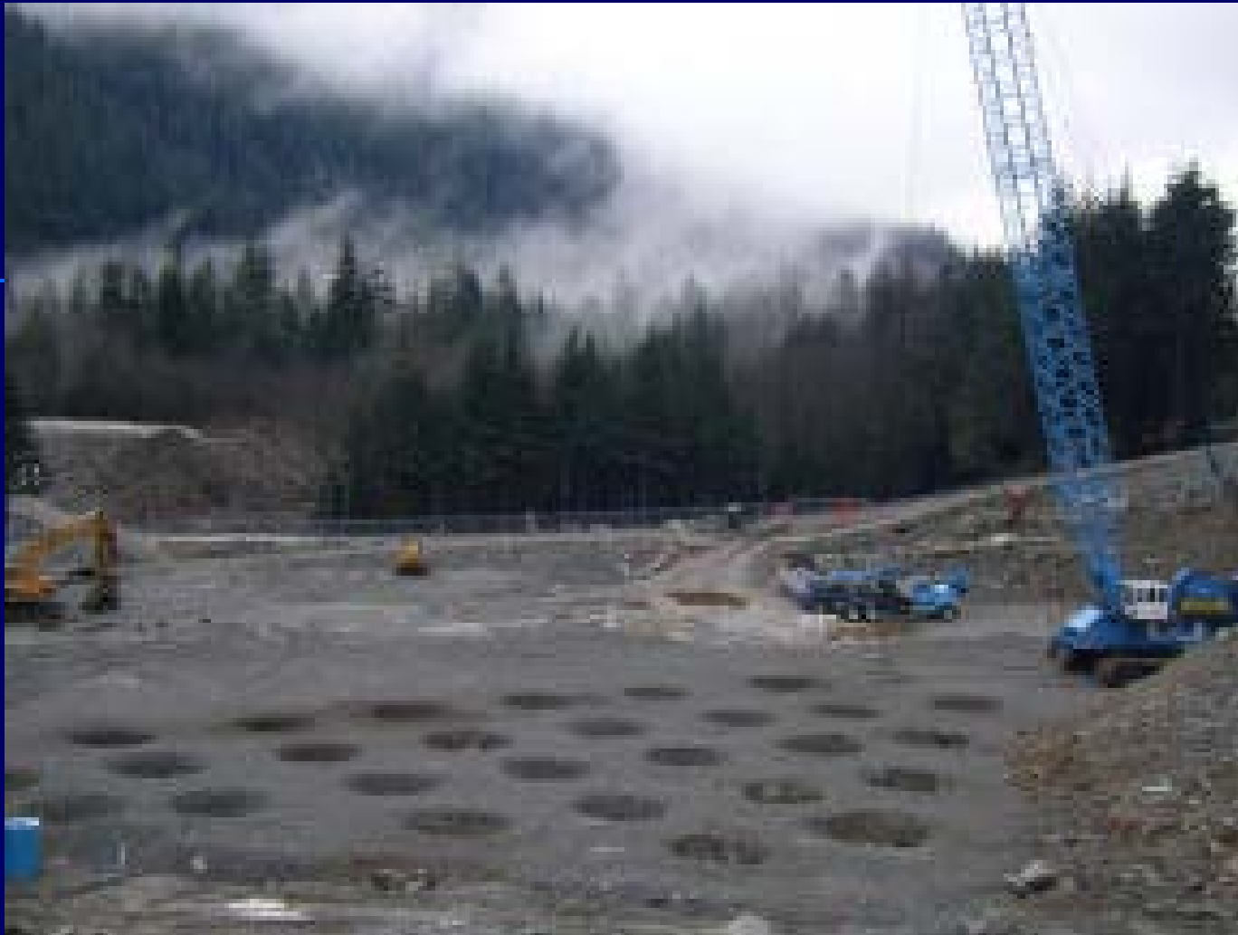
Deep Dynamic Compaction at Seymour Falls Dam Most drops were 25 tonnes from 25 meters Ave. energy was 550 tonne-m/sq m. (from Murray, et al, 2005)
