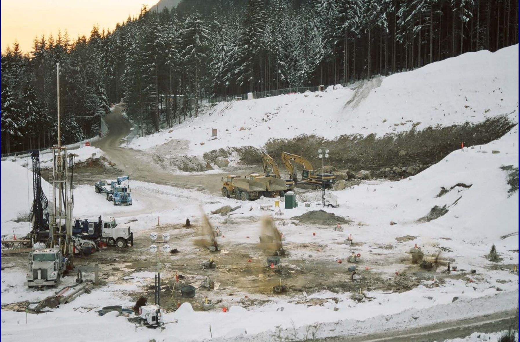
Densification of a high gravel and cobble content layer at Seymour Falls Dam, BC - note gas and water ejecting from blast holes (from Elliott, et al)
